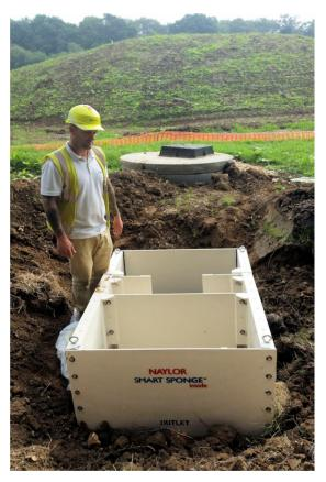
11) The Smart Sponge Smart Paks should be checked annually to see if replacement is required. This can be done simply by lifting the cage containing the units and weighing them – when the weight is double that of the installed weight then they should be replaced. Alternatively this can be done by appearance – a blackened unit that has started to turn to a gel indicates that a replacement is required.
